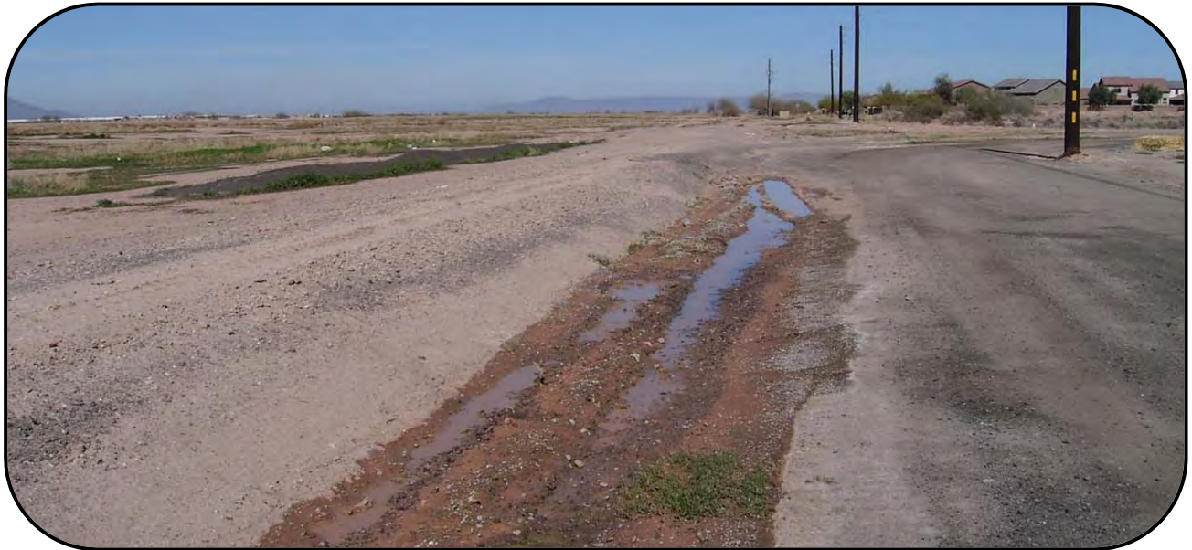
Figure 8: Water Retention in Street in Area Scheduled for Retention Basin
