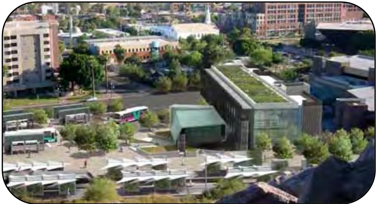
Figure 41: Tempe Transportation Center
