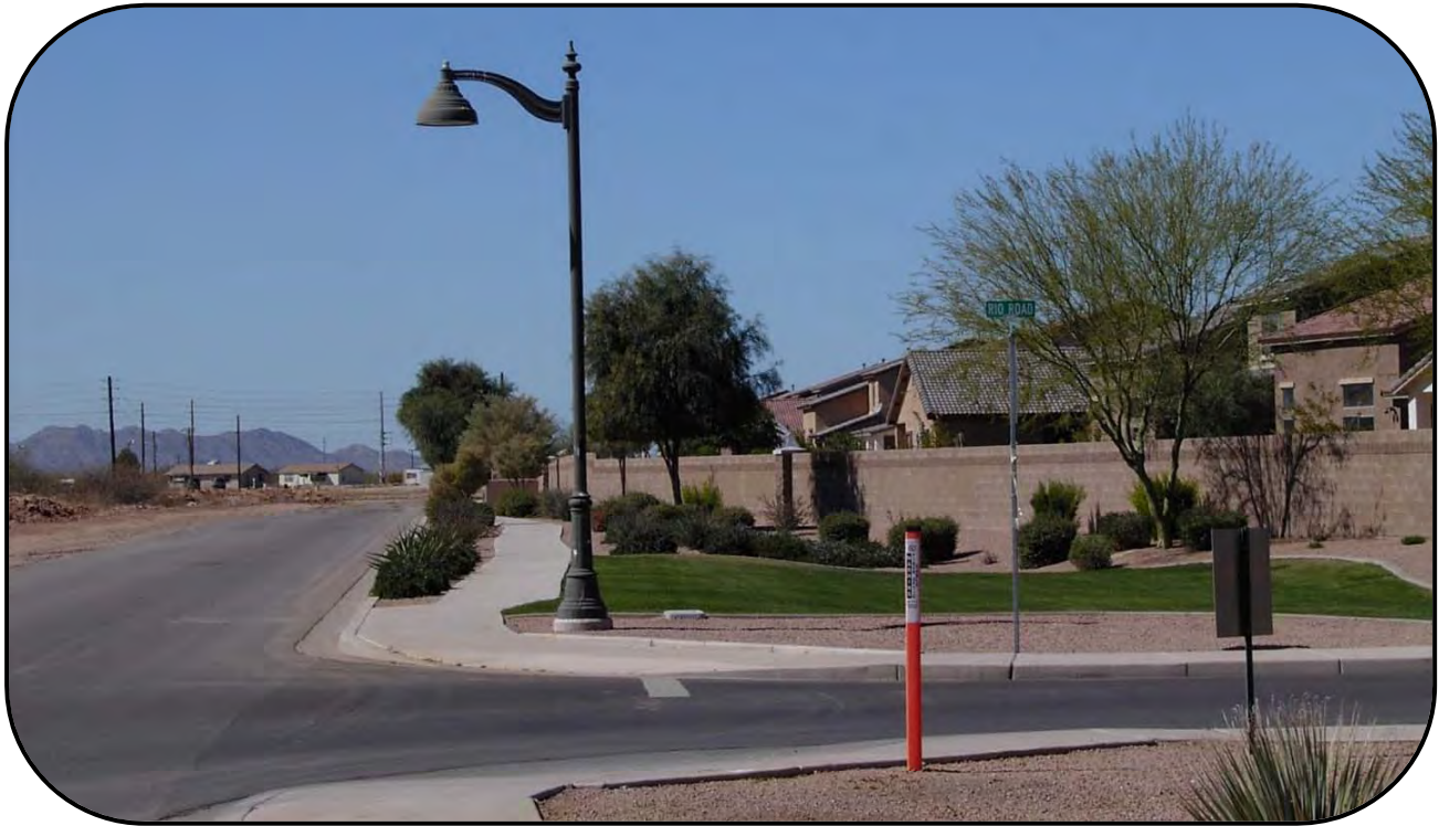
Figure 33: Edison Road Streetscape
