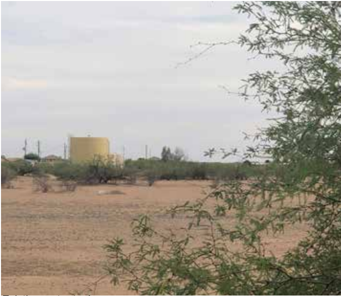
Existing water tanks
