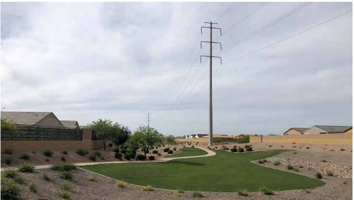
A multi-use trail should be constructed within the power transmission line easement
