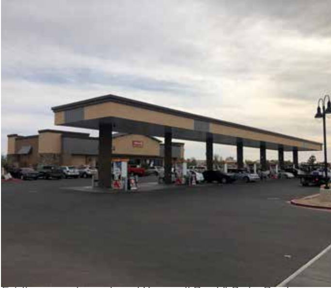
Existing convenience store at Honeycutt Road & Porter Road
