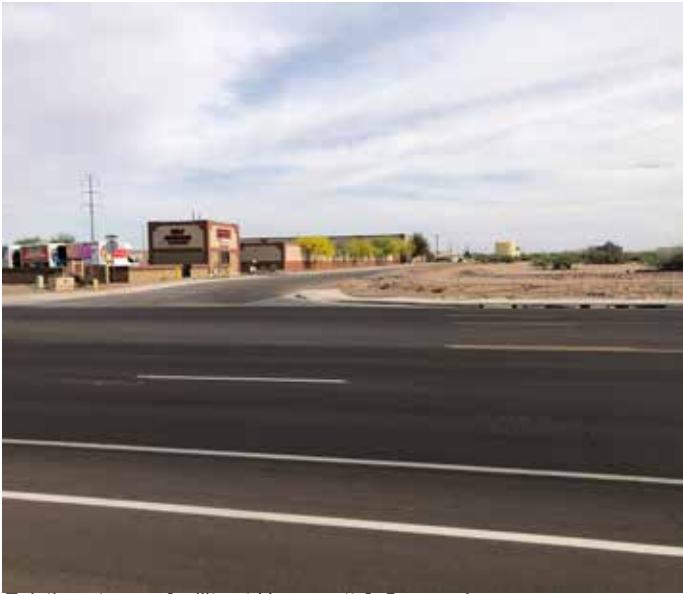
Existing storage facility at Honeycutt & Gunsmoke
